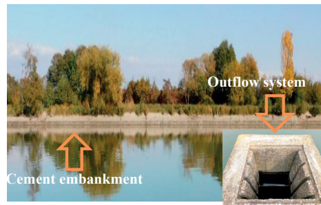
Figure 2. B.E.3 pond - Defining construction element (Original)
